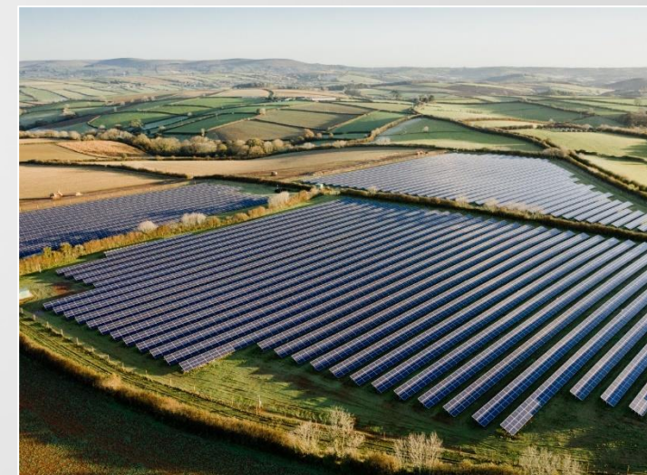
Large Scale & Project Solutions
