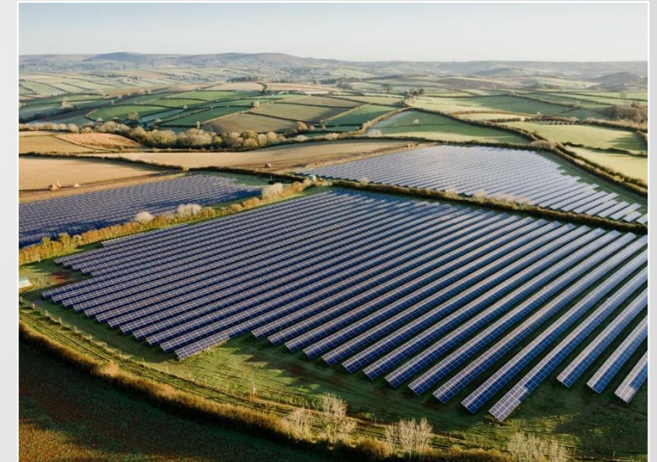
Large Scale & Project Solutions
