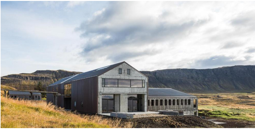
Figure 4. Drangar renovation project in Iceland. Copyright: Gallery of Drangar Renovation / Studio Granda – 2 ( archdaily.com )
